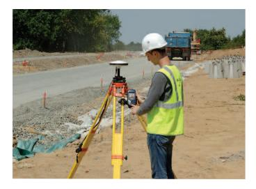
Stop & go surveys are simplified with ProMark3. The portability and the user-friendly interface enable a one-man crew to perform quick and reliable surveys.
